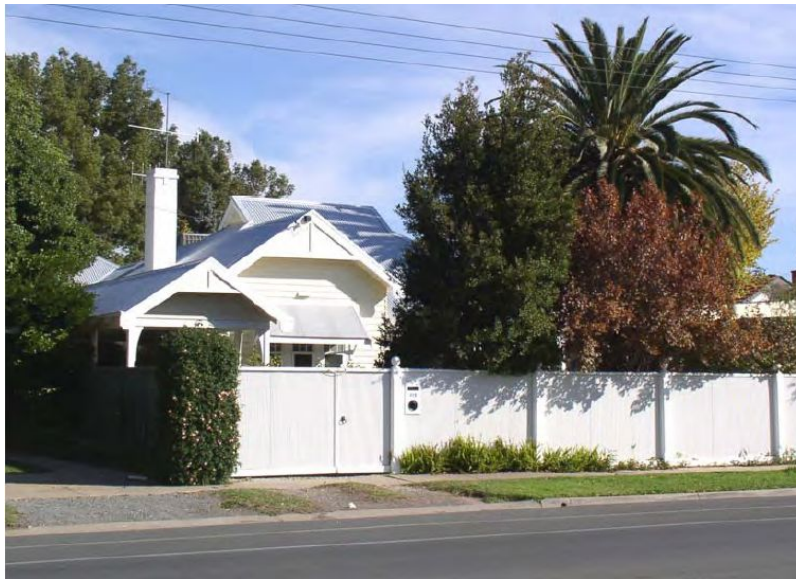
House at 112 Knight Street, Shepparton
