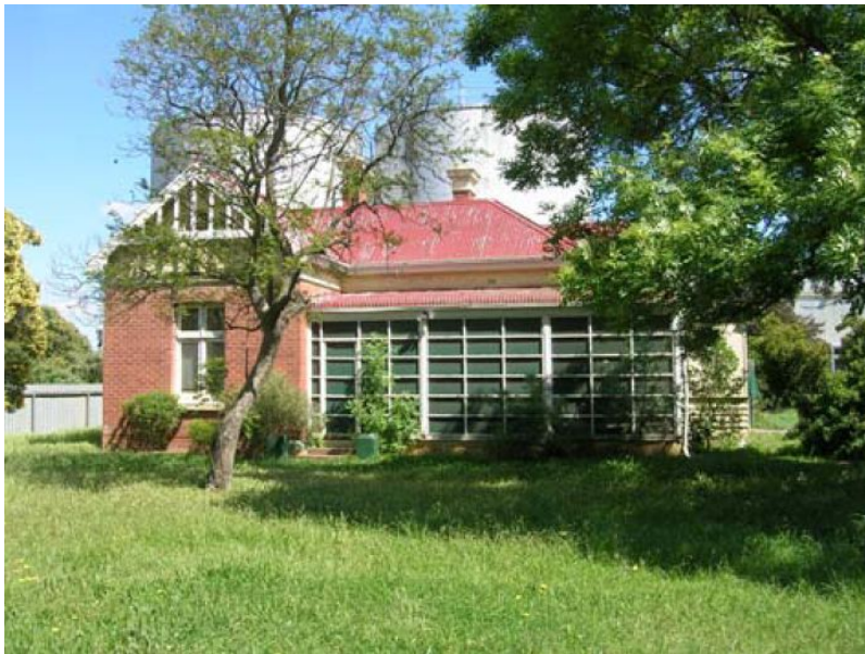
Residence at 2 Archer Street, Mooroopna
