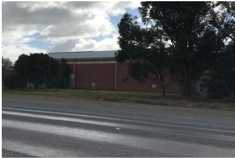
6455 Midland Highway, Ardmona (Dundas Simson Coolstore)
