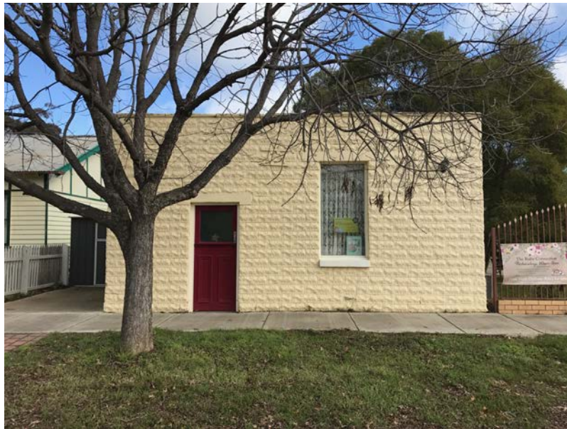
114-120 Waverley Avenue, Merrigum (office)
