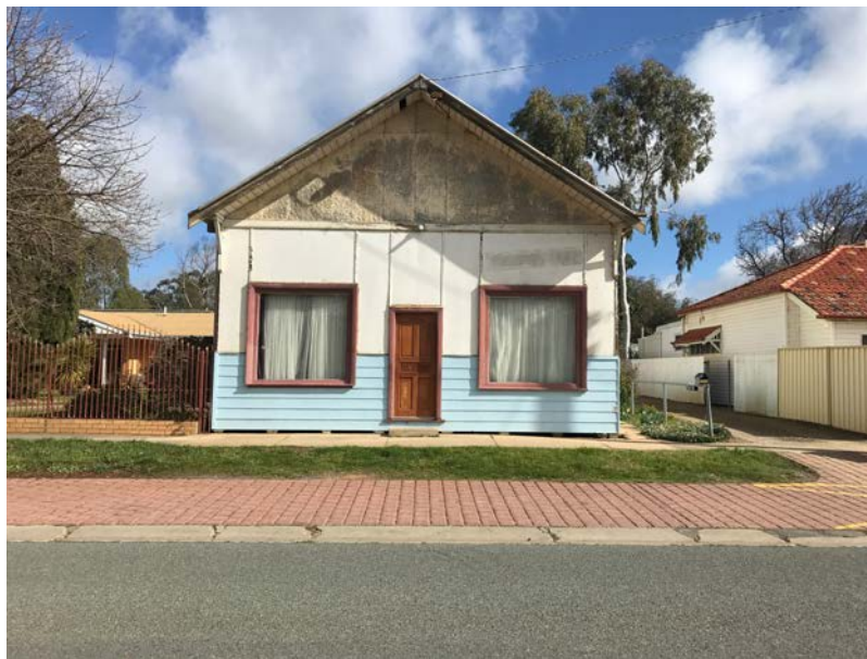
122 Waverley Avenue, Merrigum (former Billiard Parlour)
