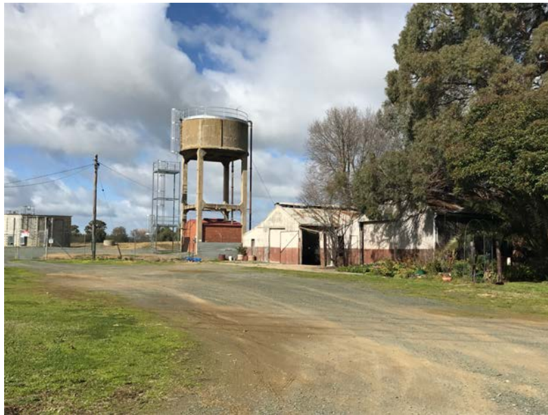
104-108 Morrissey Street, Merrigum (Water Tower)
