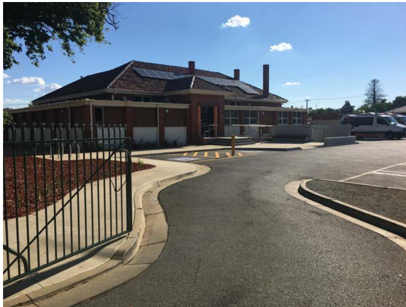
100-104 Corio Street, Shepparton (Una Hospital)
