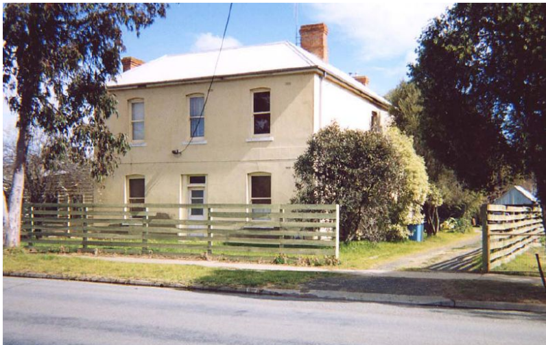
House at 88-92 Waverley Avenue, Merrigum
