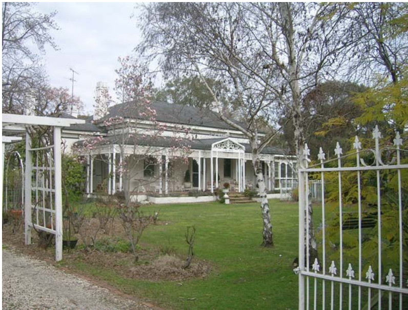
House at 22 Knight Street Shepparton
