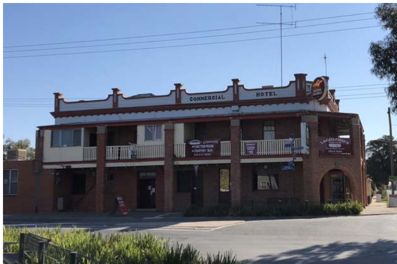
Commercial Hotel after the paint was removed from the masonry
