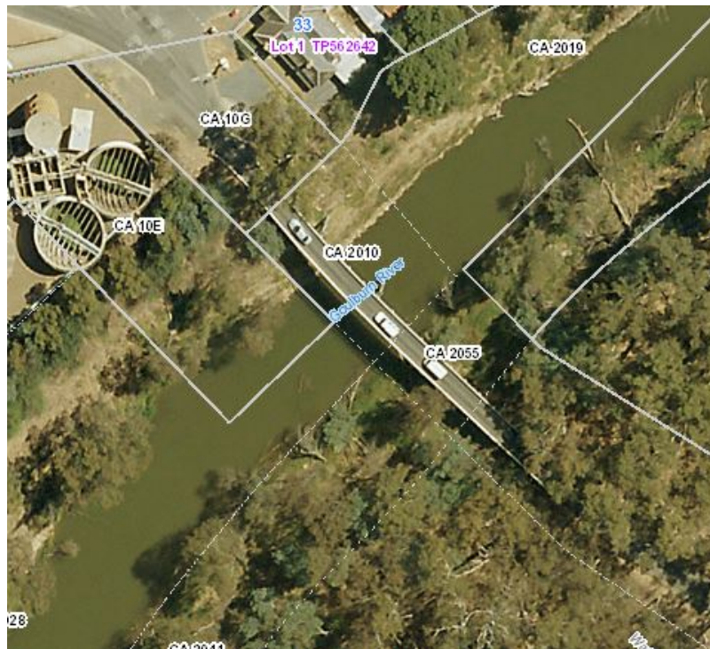
Road over Goulburn River, Watt Road, Mooroopna (Mooroopna-Kialla Bridge)
