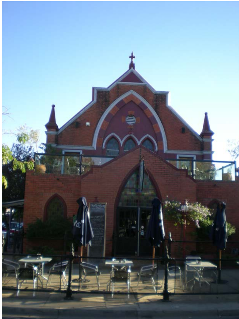
The former Baptist Church
