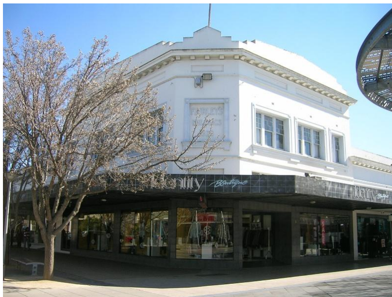
Fairley Building Fraser & Maude Streets Shepparton
