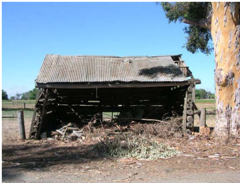
Structure 1 - Facade facing onto the laneway
