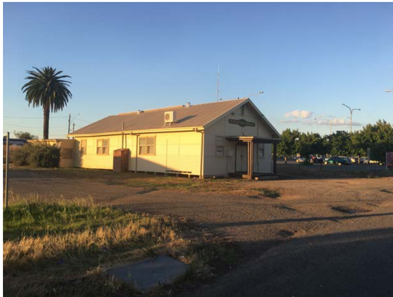
2 Purcell Street, Shepparton (VRI building)
