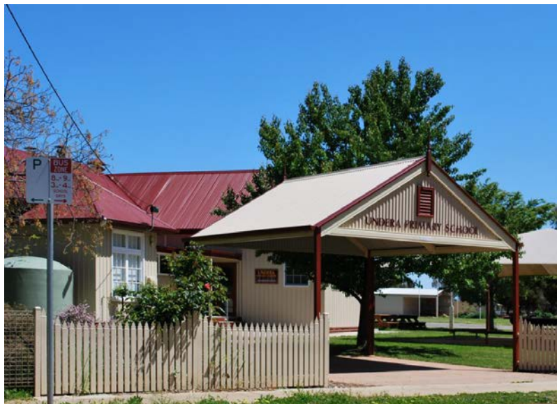
45-55 Anderson Street, Undera (Undera Primary School)
