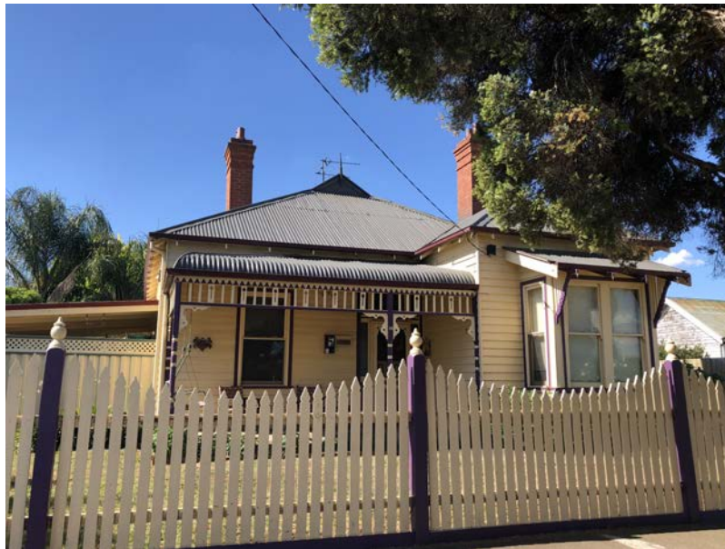
16 Alexandra Street, Mooroopna (former Methodist Parsonage)
