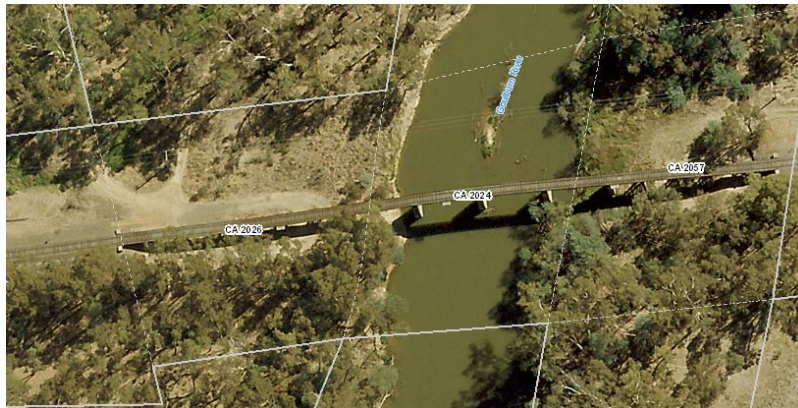
Mooroopna Rail Bridge, Mooroopna
