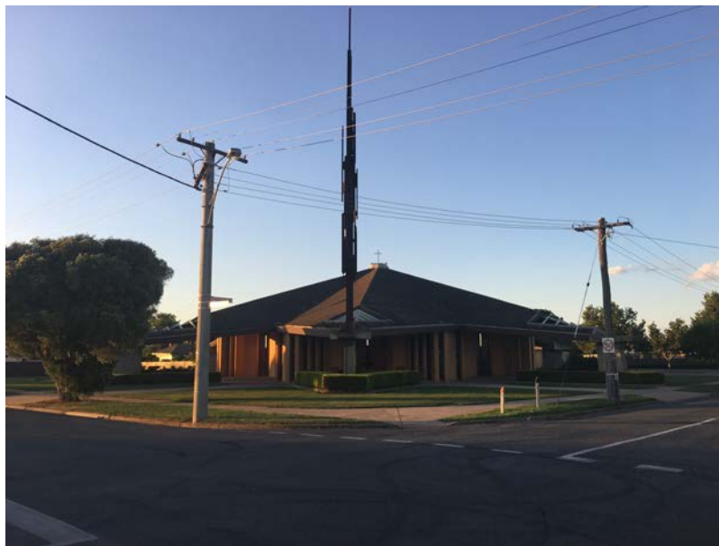
18-22 Hamilton Street, Shepparton (St Mel's Catholic Church)
