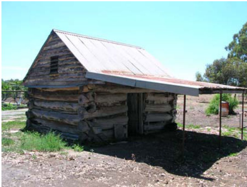
South facade - showing skillion verandah
