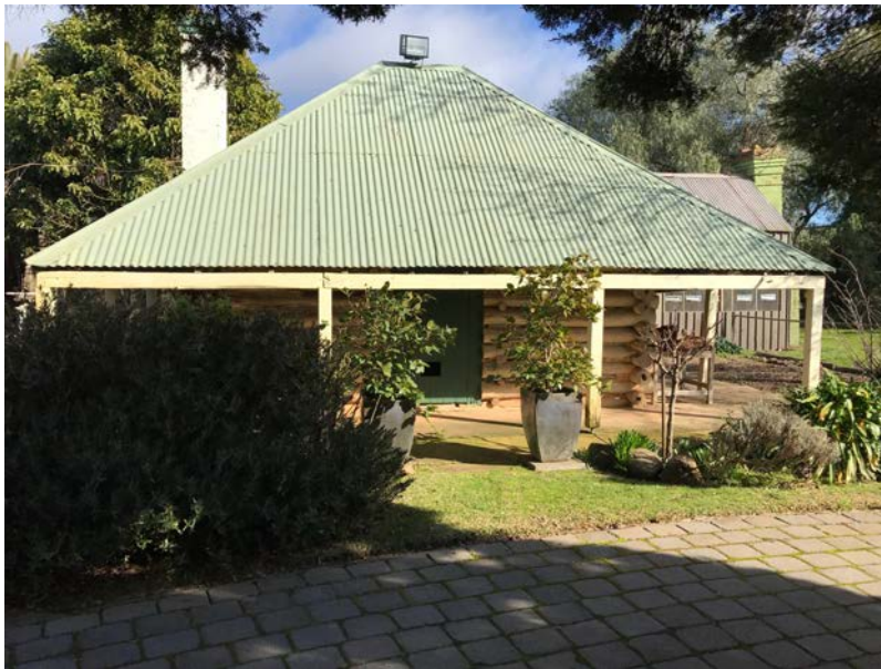
230 Manley Road, Mooroopna North West (Kelso Park - Ryan's Log Building)
