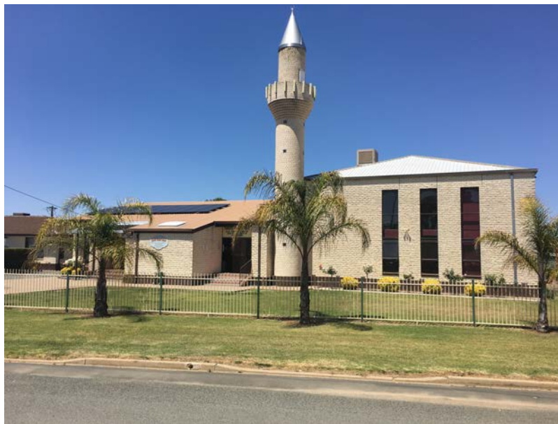
209-231 McLennan Street, Moorroopna (Turkish Mosque)
