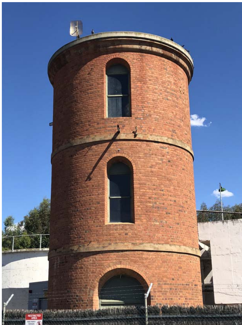
35 McLennan Street, Mooroopna (Brick Water Tower)
