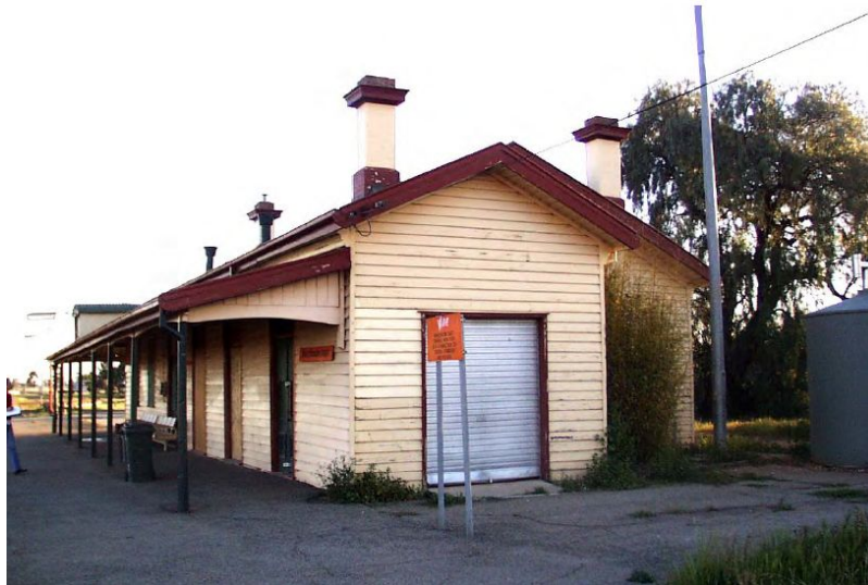
Murchison East Railway Station
