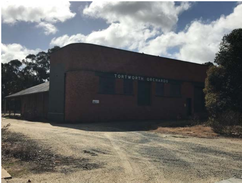
113-117 Morrissey Street, Merrigum (the former Merrigum Butter Factory)
