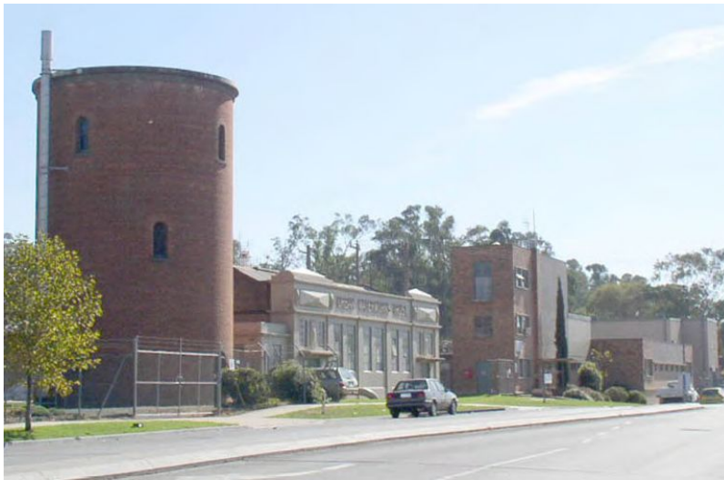
Waterworks building and tower
