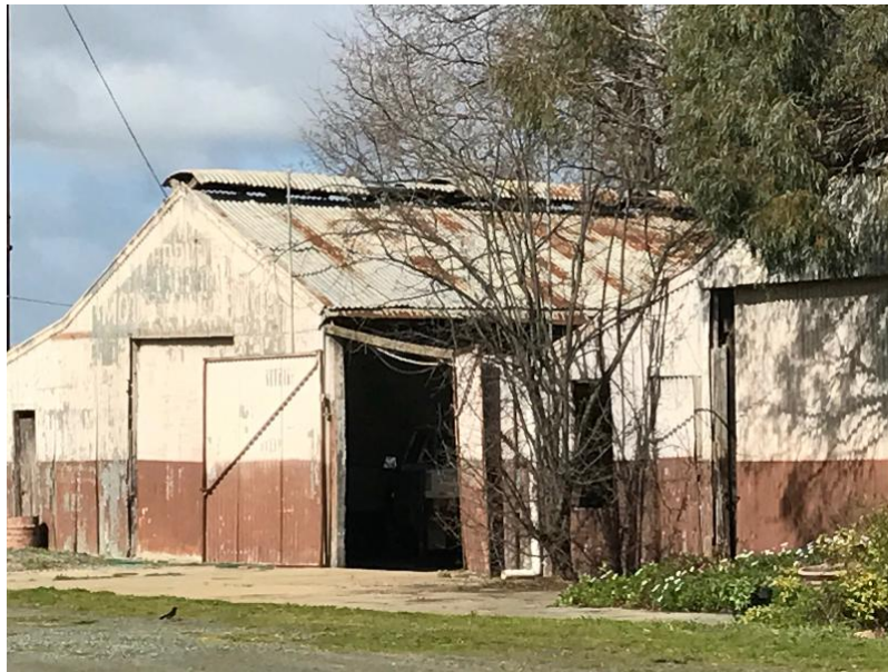
102 Morrissey Street, Merrigum (Blacksmith and Motor Garage)
