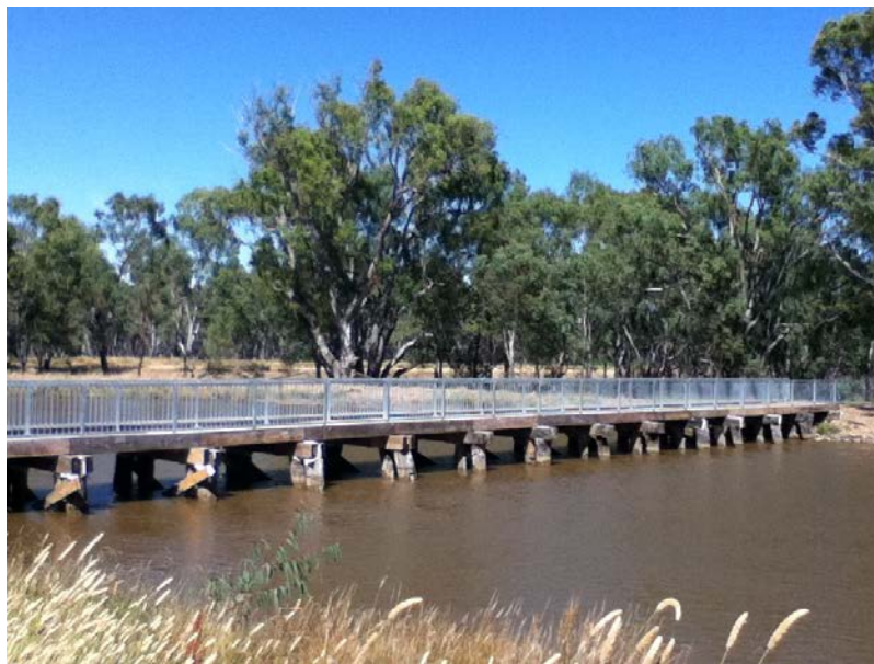
Rail Bridge over the Stuart-Murray Canal
