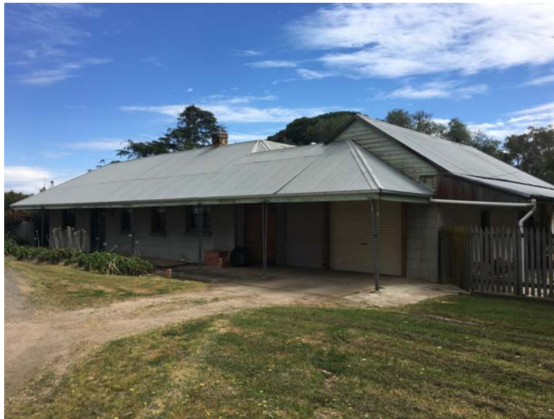
5475 Goulburn Valley Highway, Moorilim
