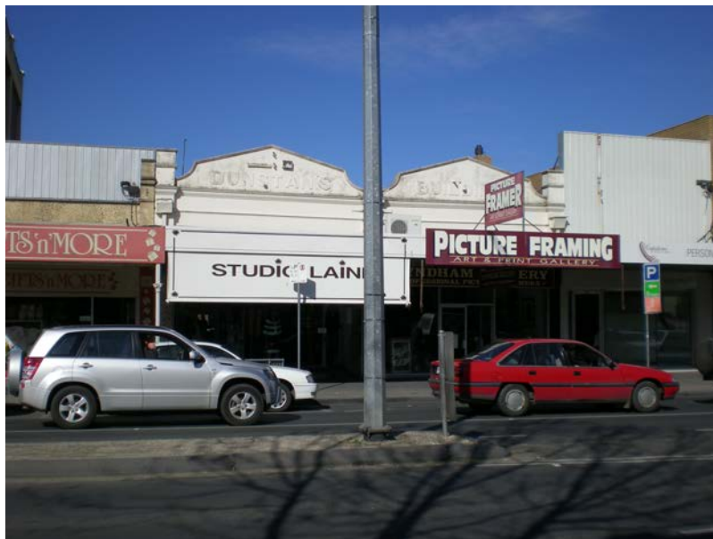
Dunstan Buildings, 337 - 339 Wyndham Street, Shepparton
